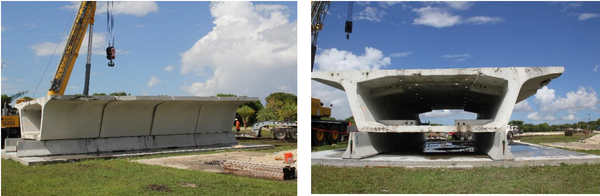
Figure 4: Segments of segmental concrete bridge at FIU.
