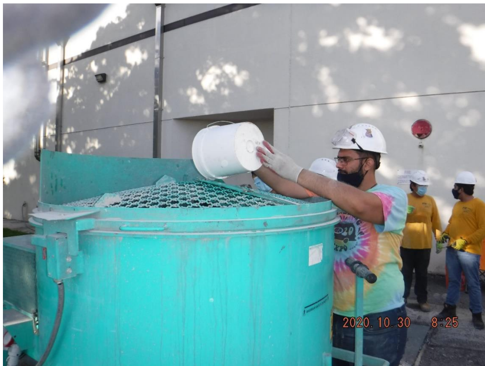
Figure 30. UHPC batching and mixing operation.
