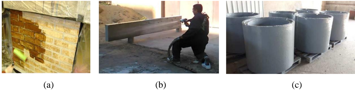
Figure 1: Application of polyurea coating (a) masonry slab (photo is taken from [4]), (b) RC beam specimens (photo is taken from [3]), and (c) concrete pipe (photo is taken from [5]).
