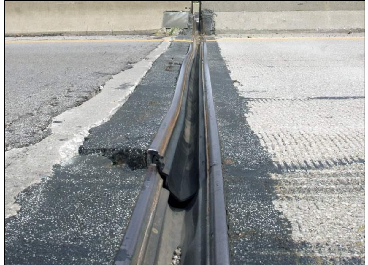
Offset of deck slabs and damage to joint seal
