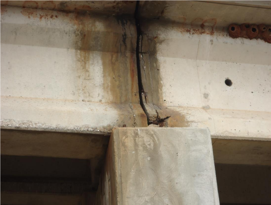
Spalling and discoloration of prestressed beam ends
