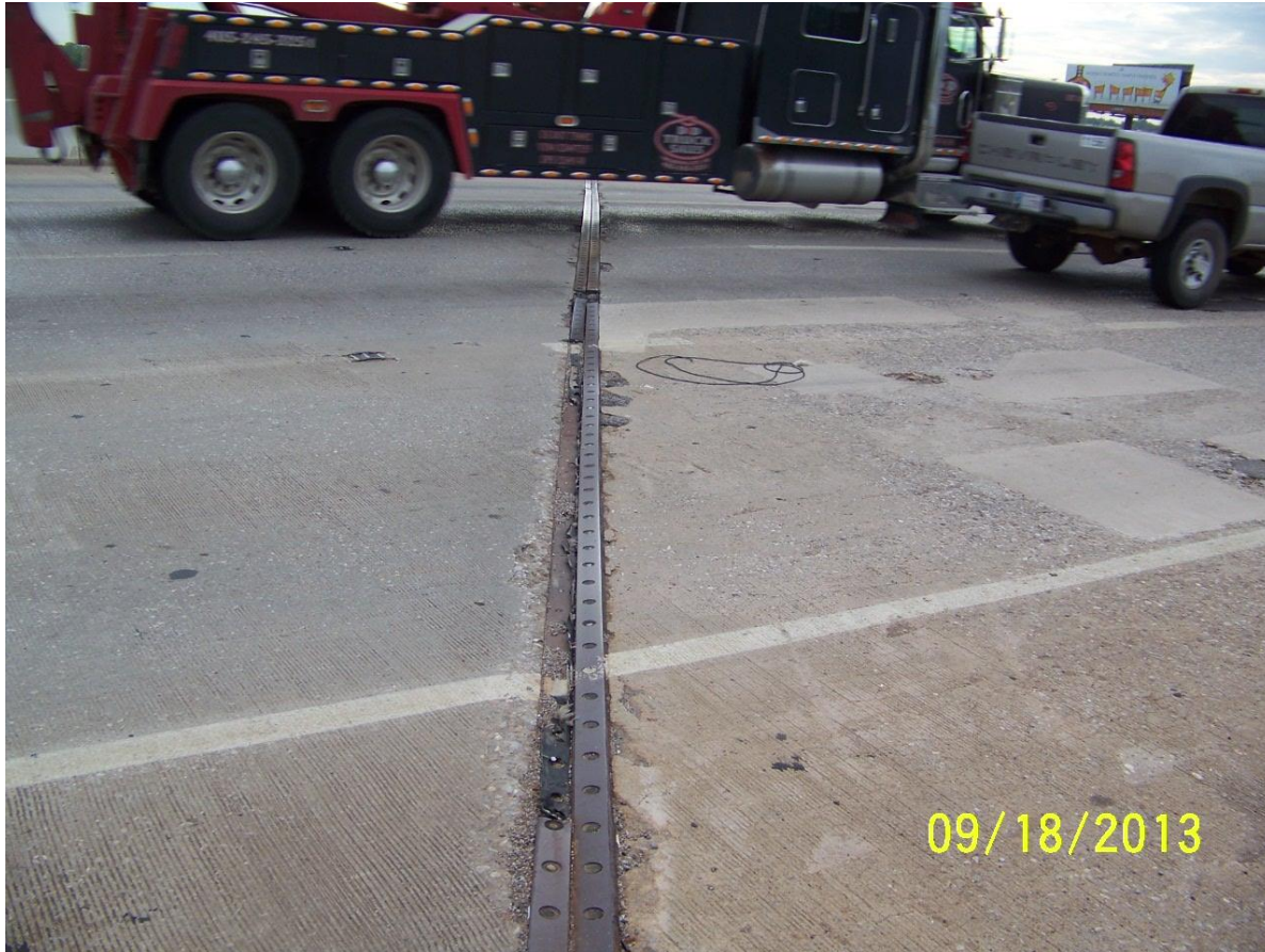
Spalling and loss of steel armoring Photo curtesy of Walt Peters
