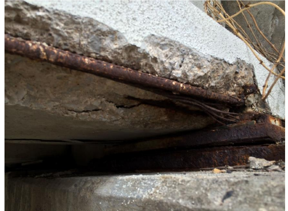
Close-up of corrosion induced spalling
