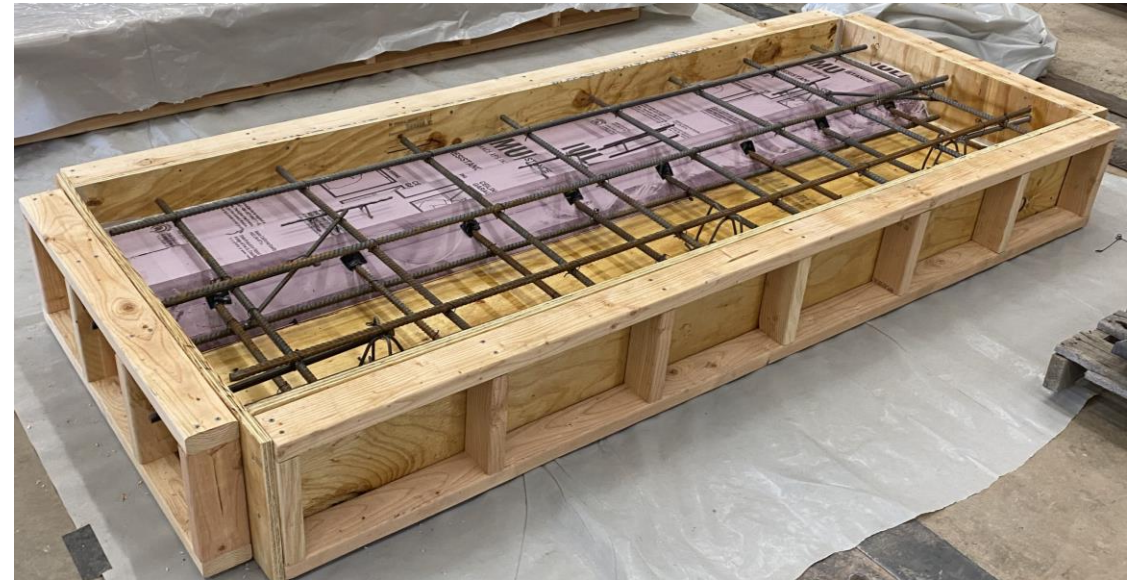
Formwork for connected panel with installed rebar
