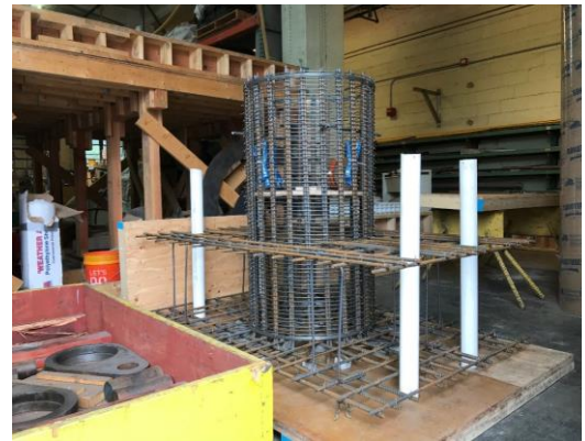
Figure 2. Photo of Shaft and Base Reinforcement
