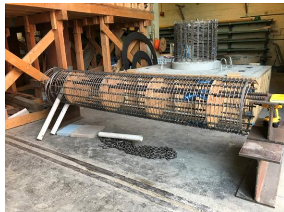
Figure 4. Photo of Column Reinforcement Cage
