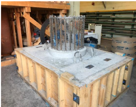
Figure 3. Photo of Shaft Reinforcement and Cast Base
