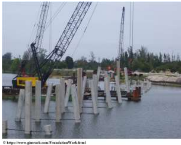
Figure 7: Prestressed-Precast Concrete Piles in marine environment
