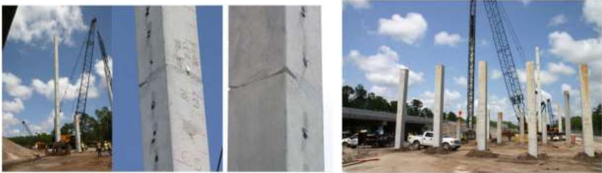
Figure 33: Pile driving using spliced pile specimen (Mullins & Sen, 2015)
