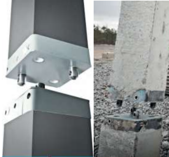
Figure 21: ABB splice
