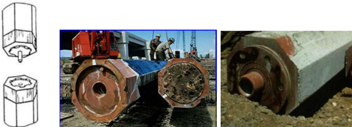
Figure 20: Mechanical splice (Mullins & Sen, 2015)
