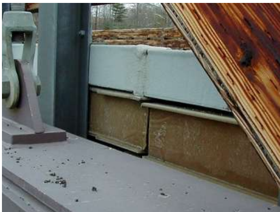
DISPLACEMENT OF FRP DECK
