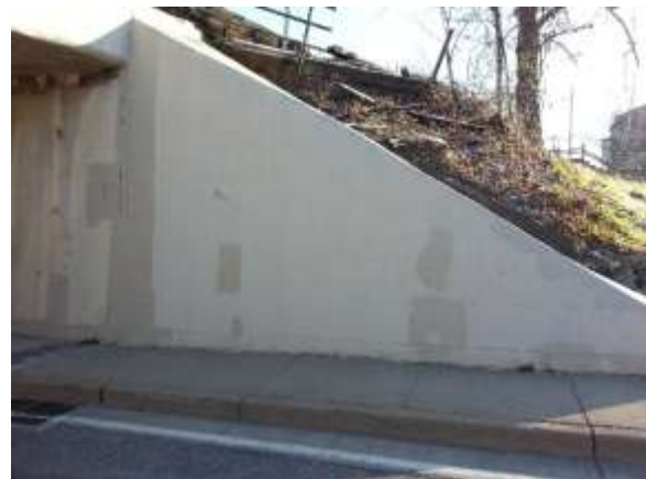
WINGWALL REPAIRED WITH FRP WRAPS
