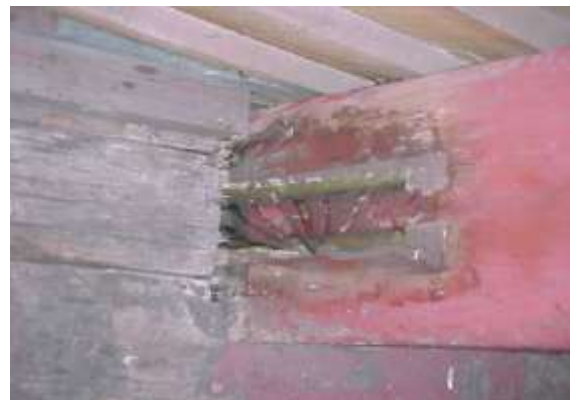
EPOXY GROUTED GFRP REINFORCEMENT
