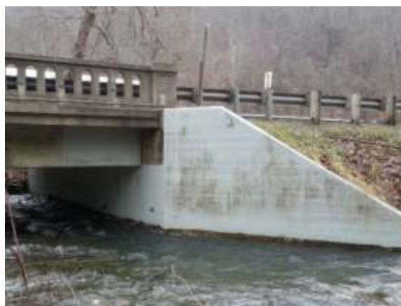
FRP WRAP ON WINGWALL AND T-BEAM
