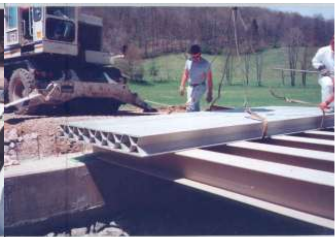
INSTALLATION OF DECK PANELS
