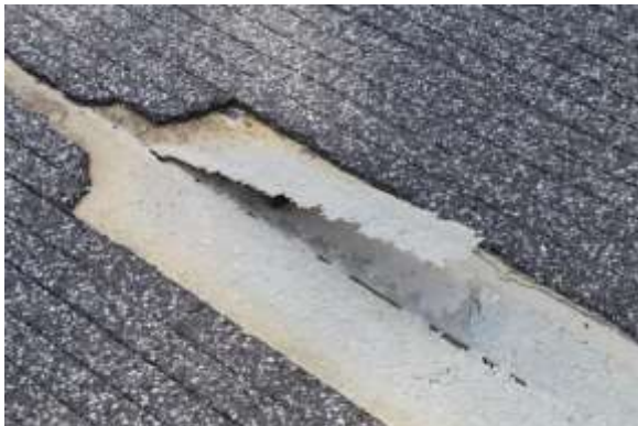
BREAK UP OF WEARING SURFACE AND DETERIORATION OF DECK PANEL JOINT REINFORCEMENT
