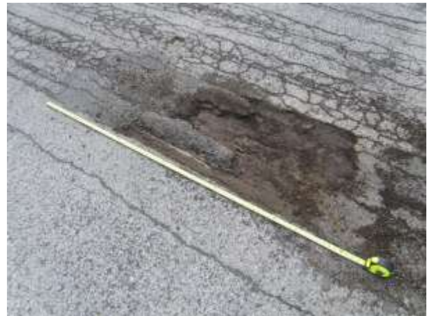
MISSING ASPHALT AT ABUTMENT 2
