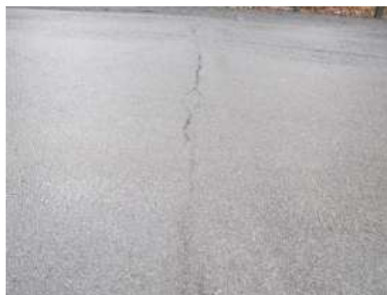
TYPICAL TRANSVERSE CRACKING
