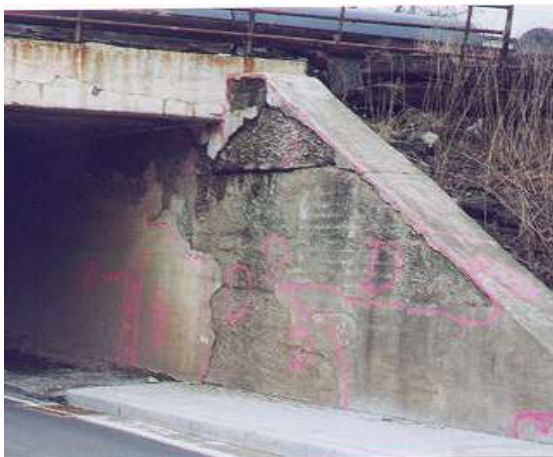
WINGWALL PRIOR TO REHABILITATION
