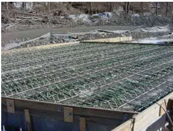
GFRP REBAR IN DECK
