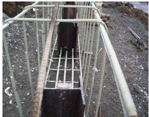
CLOSE UP OF REBAR IN ABUTMENT
