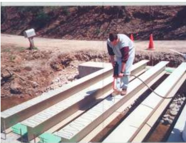
APPLICATION OF PLIOGRIP ADHESIVE TO GFRP BEAMS
