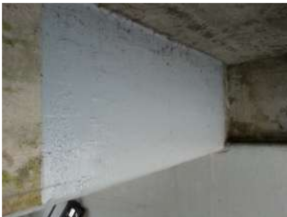
FRP ON END OF T-BEAM
