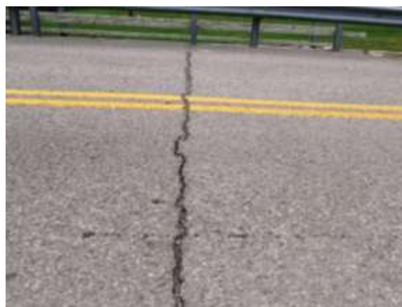
WEARING SURFACE CRACK
