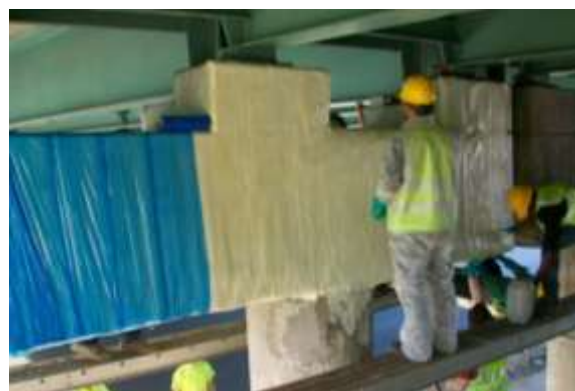
INSTALLATION OF THE FRP WRAP
