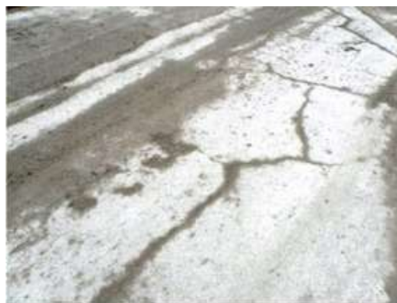
MAP CRACKING IN DECK
