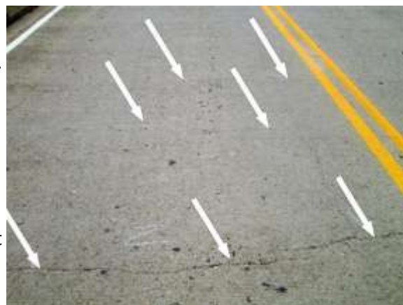
CRACKS IN THE WEARING SURFACE
