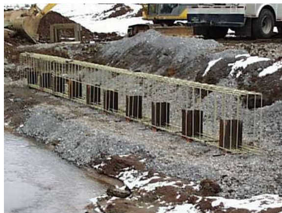
GFRP REINFORCEMENT IN ABUTMENTS
