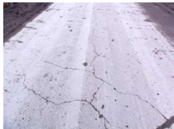
DECK CRACKING
