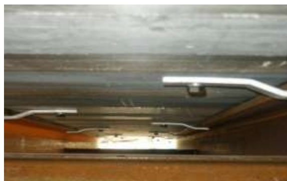
Z-CLIPS ATTACHING DECK TO BEAMS
