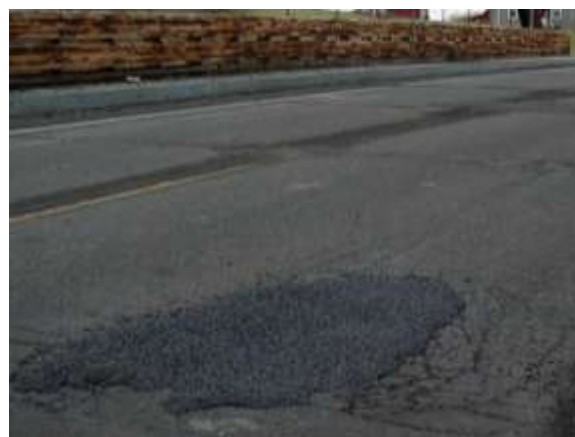
PATCHES IN WEARING SURFACE DUE TO FRP DECK FAILURE
