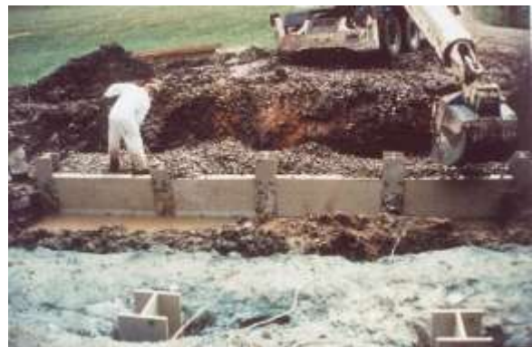
GFRP PILES/CELLULAR LAGGING MODULES
