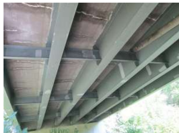
UNDERSIDE OF DECK WITH CRACKS/EFFLORESCENCE
