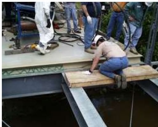
PLIOGRIP FOR DECK TO DECK CONNECTION
