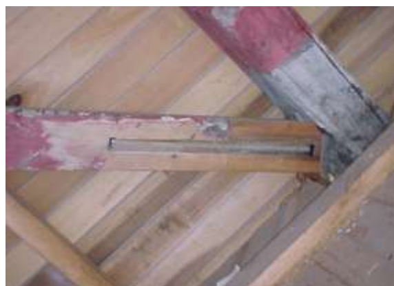
GFRP ROD EMBEDDED INTO DIAGONAL MEMBER
