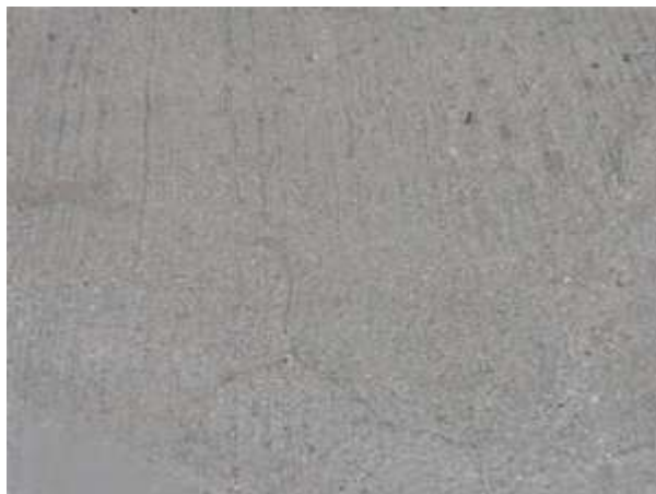
MAP CRACKING IN DECK
