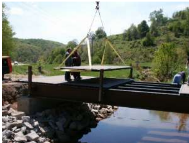
PLACEMENT OF DECK PANEL
