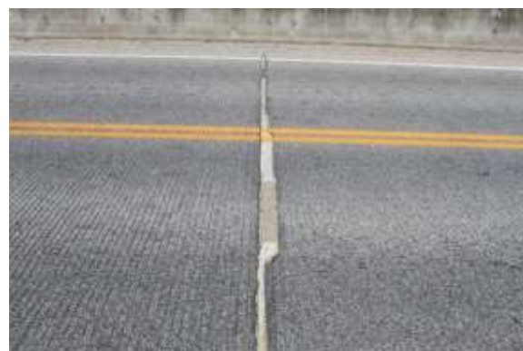
BREAKUP OF DECK PANEL JOINT
