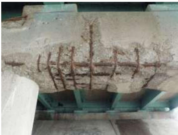
CONCRETE DETERIORATION PRIOR TO REPAIR
