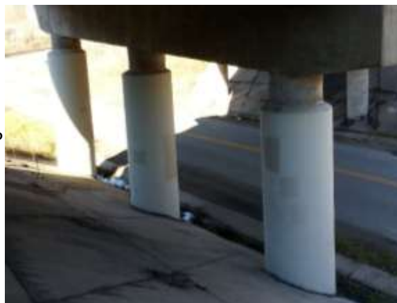
COLUMNS WRAPPED WITH FRP
