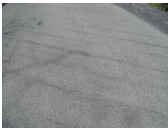
TRANSVERSE CRACKING IN WEARING SURFACE
