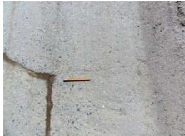
HAIRLINE CRACKS IN DECK
