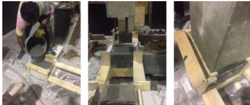
Figure 12- Construction of the Specimen 2 with shear key and dowels.
