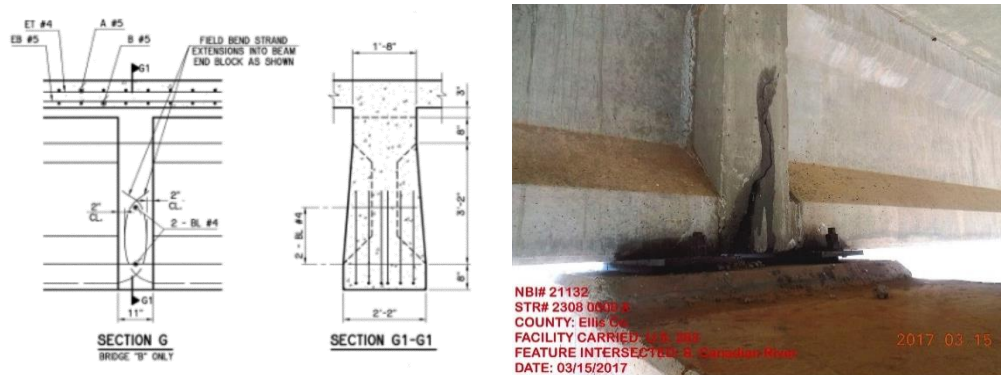
Figure 1. Detail for a typical continuity linkage block used in Oklahoma (left) and photo of a linkage block exhibiting cracking from restraint induced moments (right)
