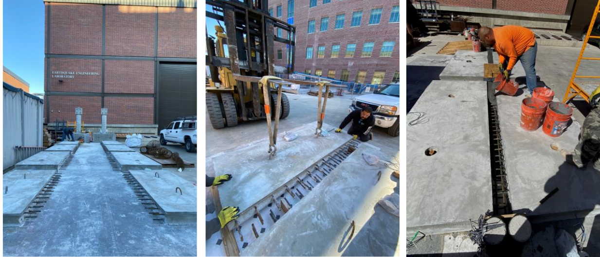
Figure 3-6: Photographs to illustrate the sequence of construction of the test specimens.
