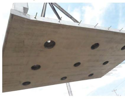
Shear Connector Pockets with Vent Holes for SCC
