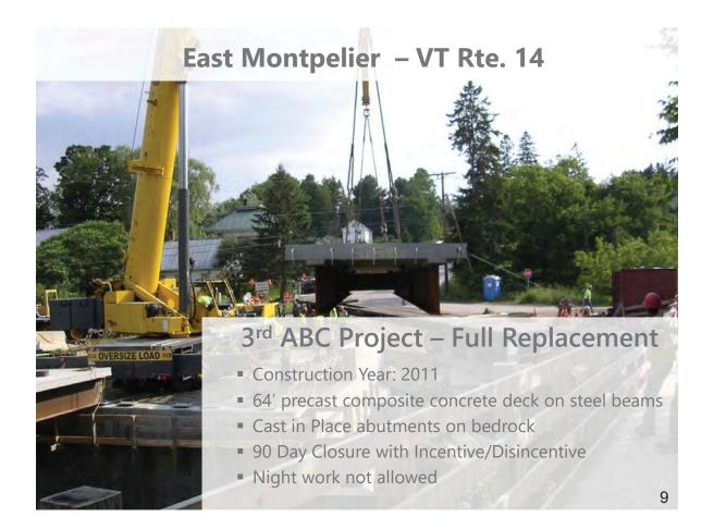
East Montpelier – Precast steel Bridge Units (PBU's)
