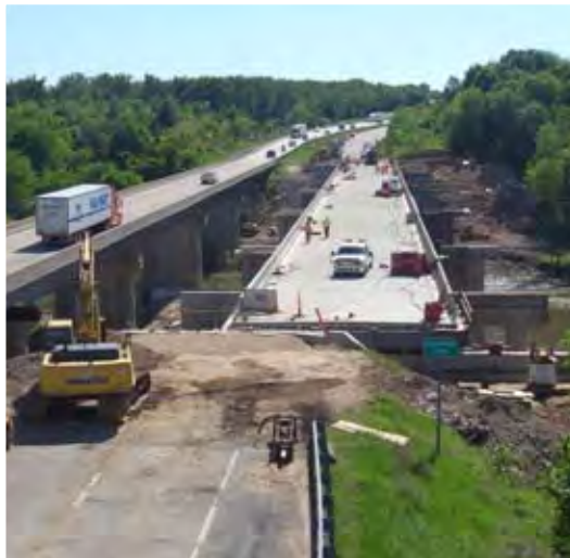
▼ 3:30 p.m.: Half-way point of the bridge move.
