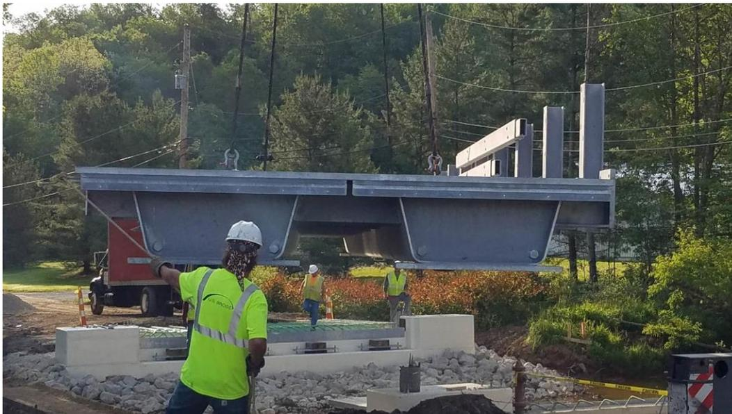
The modules were bolted together in one day. A waterproof membrane and asphalt wearing course were subsequently applied. The bridge deck was metallized with zinc on all surfaces to provide additional corrosion protection from the low pH levels of the stream. Other superstructure components were
