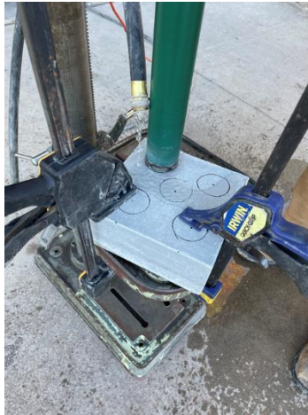
Figure 9 Core drilling using universal drilling machine
