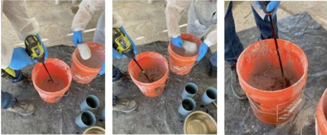
Figure 1: Polymer concrete mixing process
