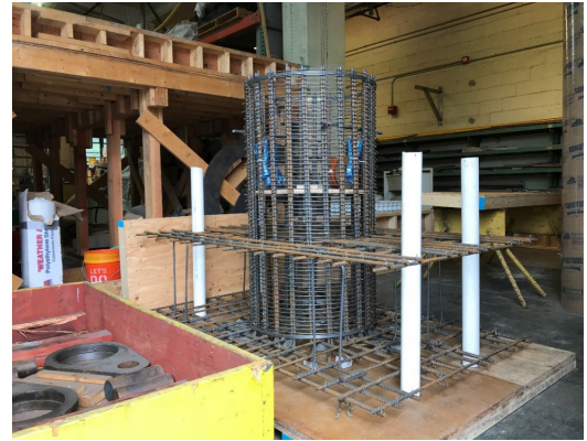
Figure 2. Photo of Shaft and Base Reinforcement
