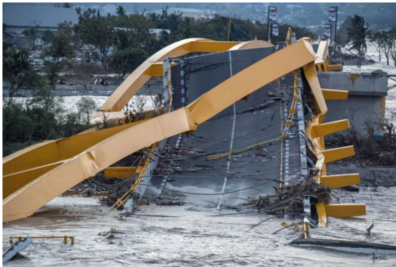
Figure 1. Ponulele Bridge Destroyed by 2018 Tsunami
