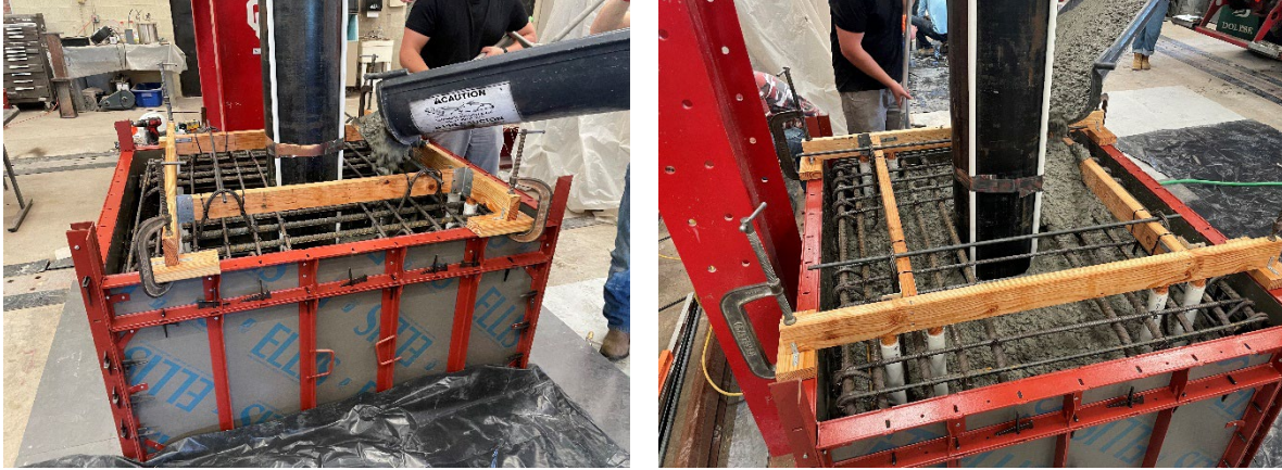
Figure 4. Fabrication of HC-FCS Column Bases with Embedded Steel Tubes
