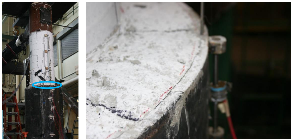
Figure 3.36 Specimen 30-21-LD Cracks at Edge of the Pile at 0.7% Drift
