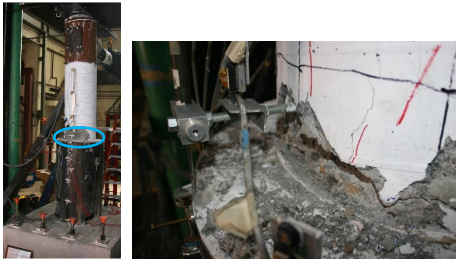
Figure 3.41. Specimen 30-21-LD Northern Column Face Spalled Region at 3.8% Drift
