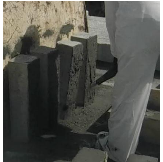
Figure 16. Horizontal Spray note Rebound
