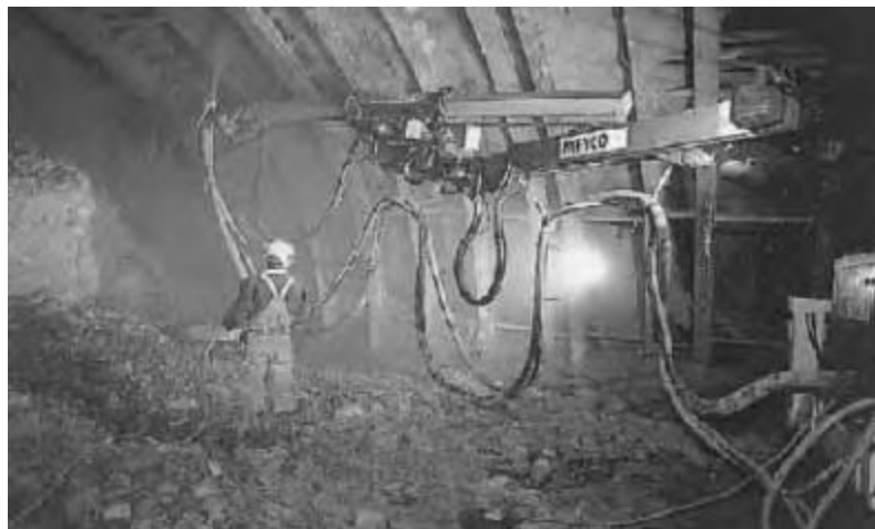
Figure 18. MEYCO Robojet Manipulator. [17]
