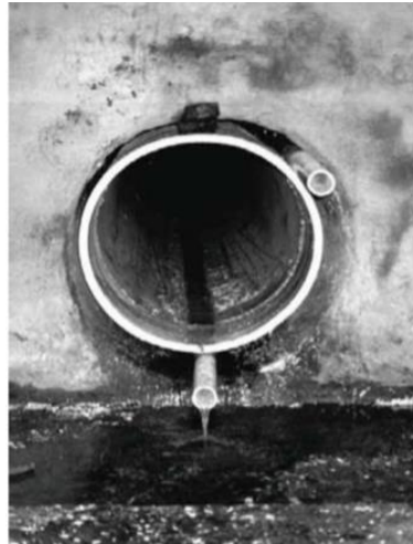
Figure 3. PVC Slip liner and Grout Injection Pipes [2]
