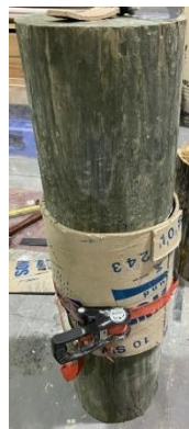
Figure 29. Construction process for partial shell encasement.
