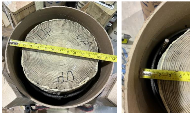
Figure 51. Uniform gap between timber and tube form.
