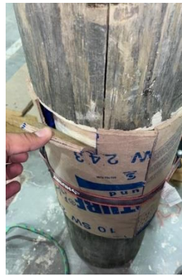
Figure 29. Construction process for partial shell encasement.
