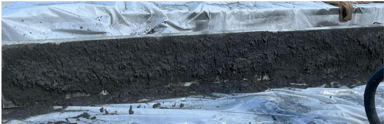
**Figure 22.** Showing the pneumatic application of UHPC, Third layer.
