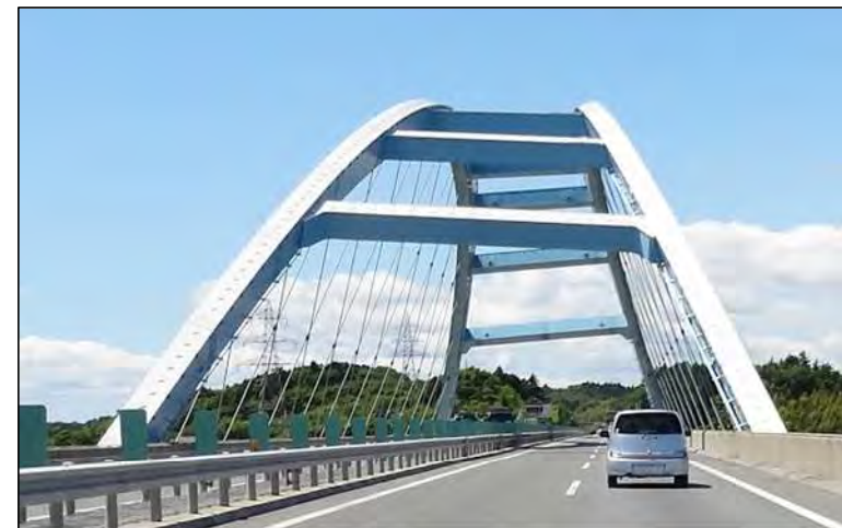
Naruse Okumatsushima Bridge, Japan
