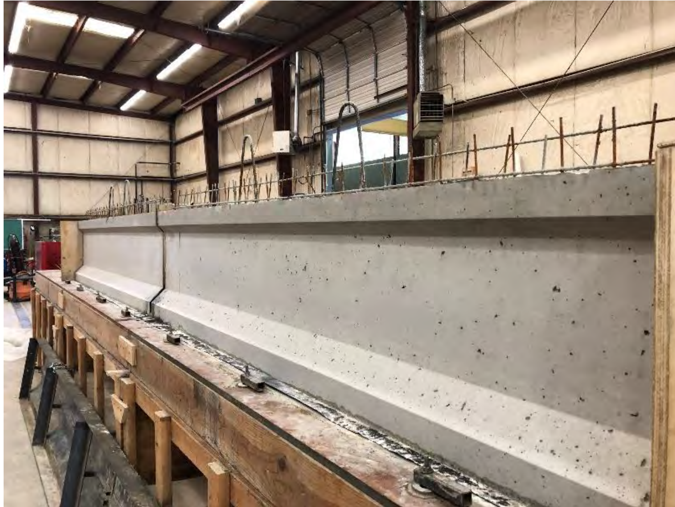
Completed girder specimens in place on the prestressing bed
