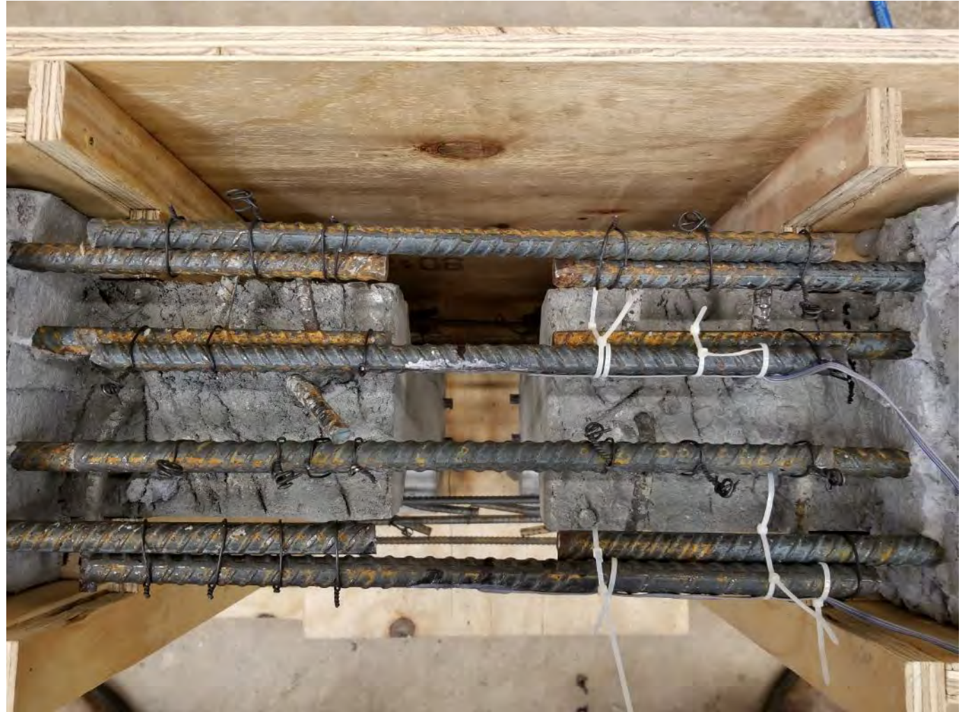
Retrofit construction continuity joint reinforcement immediately before casting
