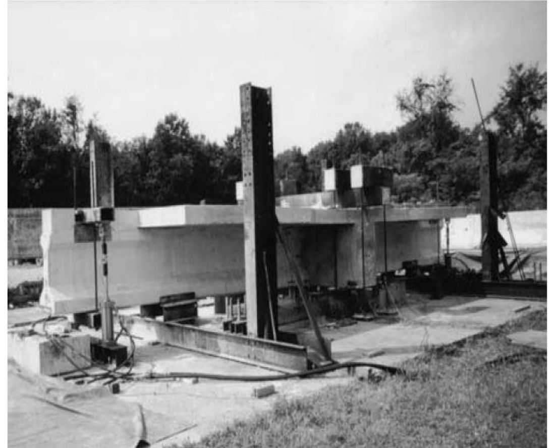
Full-scale load testing of a continuity connection by Miller (2004)
