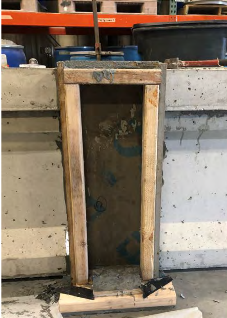
Joint formwork
