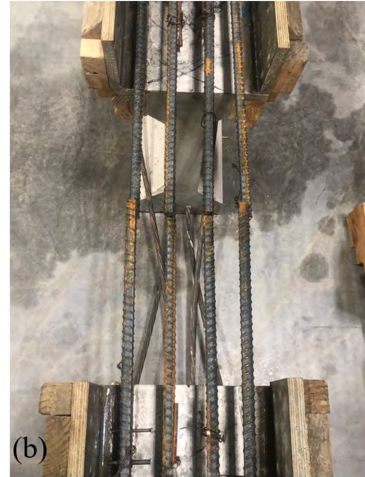
Reinforcement splice alignment
