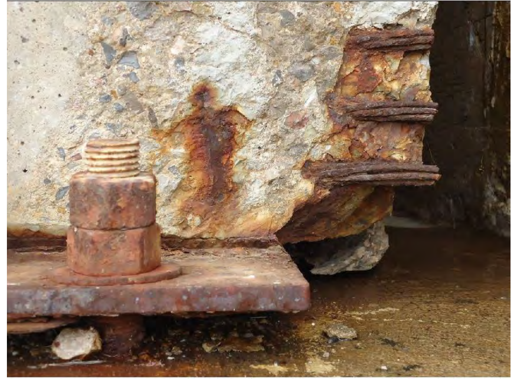
Examples of beam end deterioration in Oklahoma bridges
