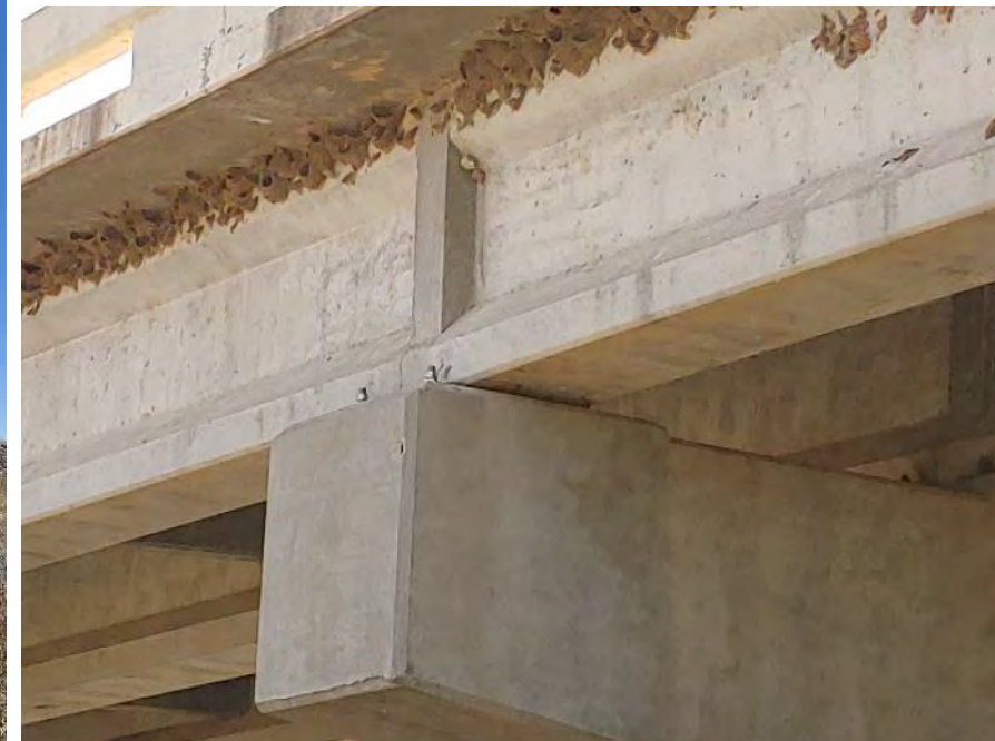
Close-up view of continuity connection
