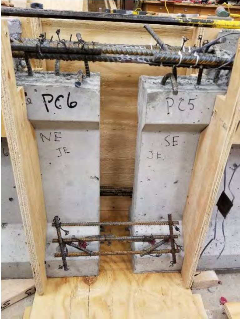
Retrofit construction continuity joint reinforcement immediately before casting
