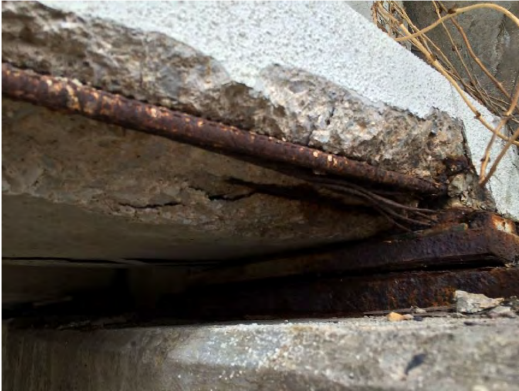
Examples of beam end deterioration in Oklahoma bridges
