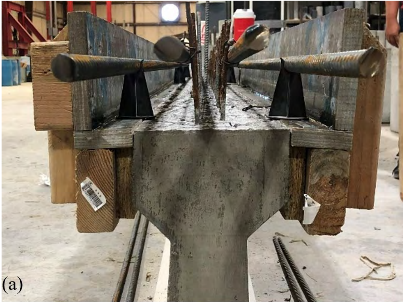
Deck reinforcement in place for casting
