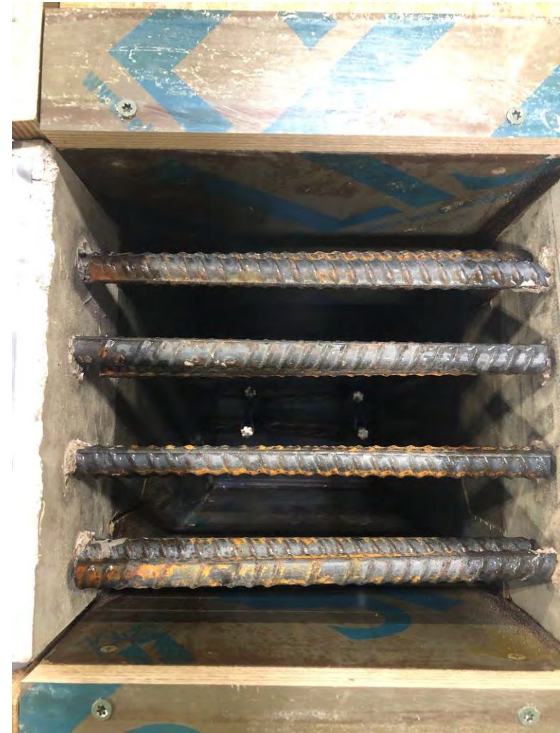
Deck reinforcement splice
