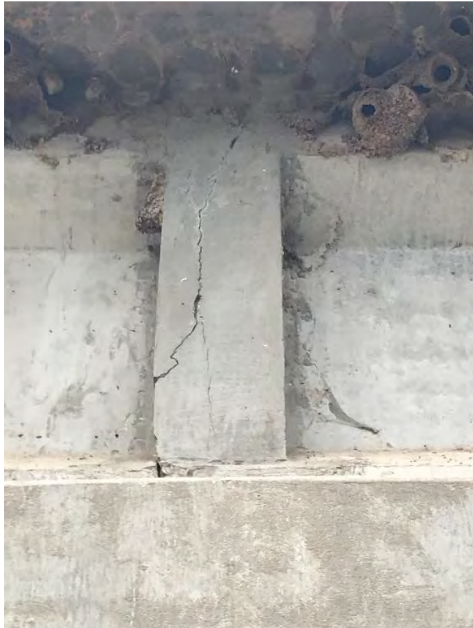
Cracking in continuity connections on U.S. 183/412 Bridge over Wolf Creek, Fort Supply, OK
