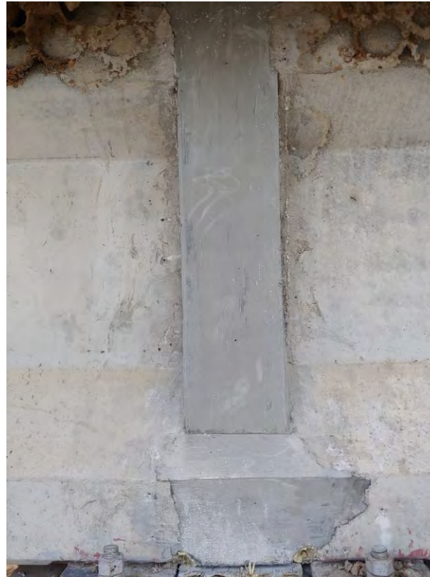
Completed UHPC joint
