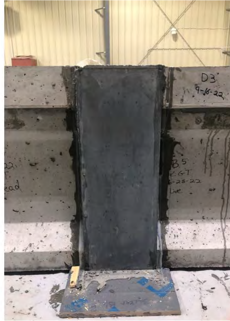
Completed UHPC connection
