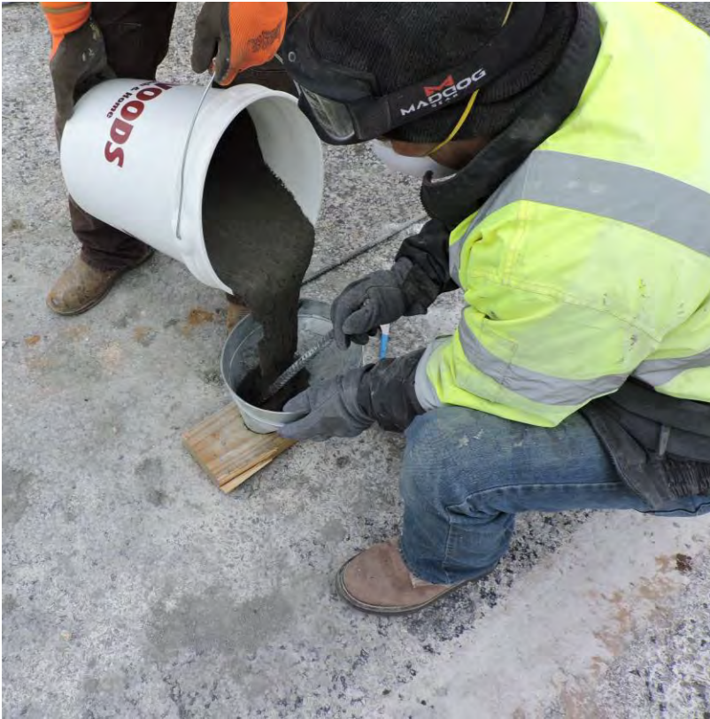
UHPC Placement through the deck
