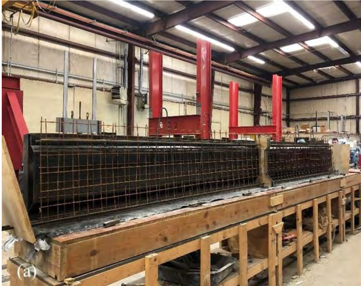
Beam formwork and reinforcement in place on the prestressing bed
