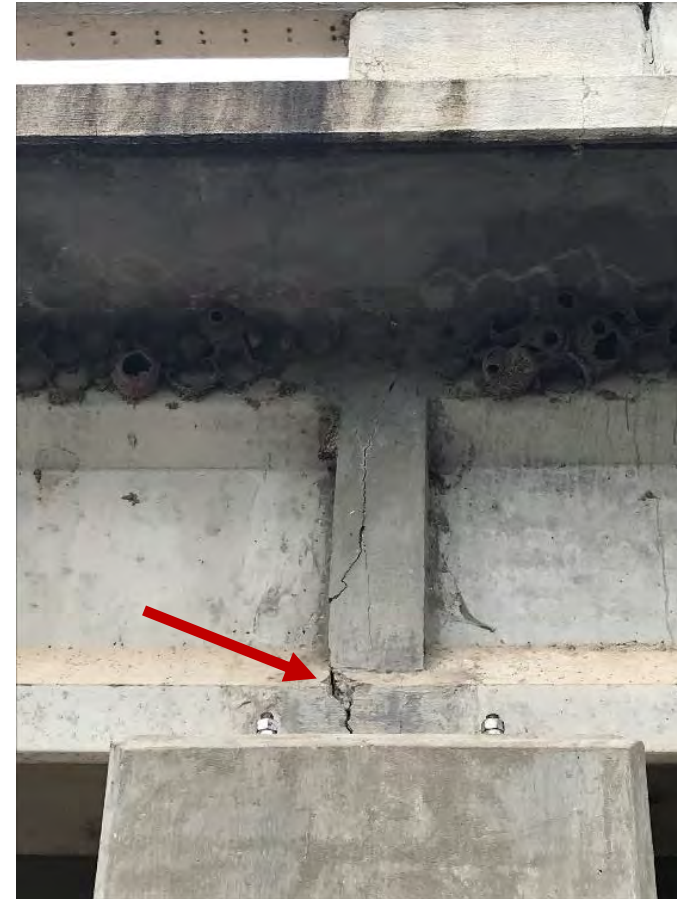
Cracking in continuity connections on U.S. 183/412 Bridge over Wolf Creek, Fort Supply, OK
