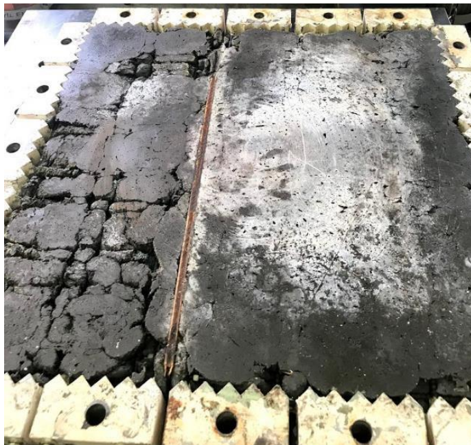
Figure A.6: Panel with poor consolidation
