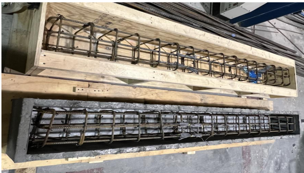
Figure 10: Reinforcement a) 3D-printed beam shell b) Corresponding conventional concrete beam
