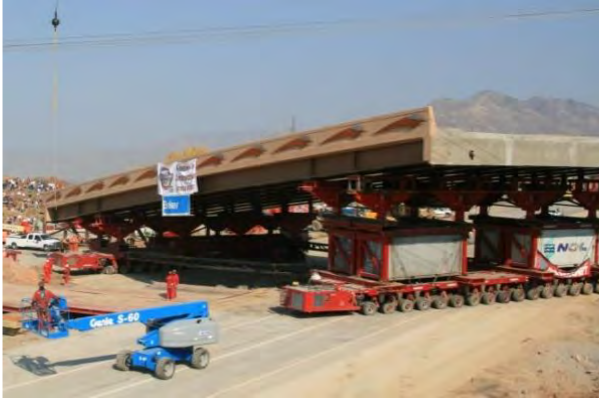
4500 South over I-215 Bridge Replacement CMGC
