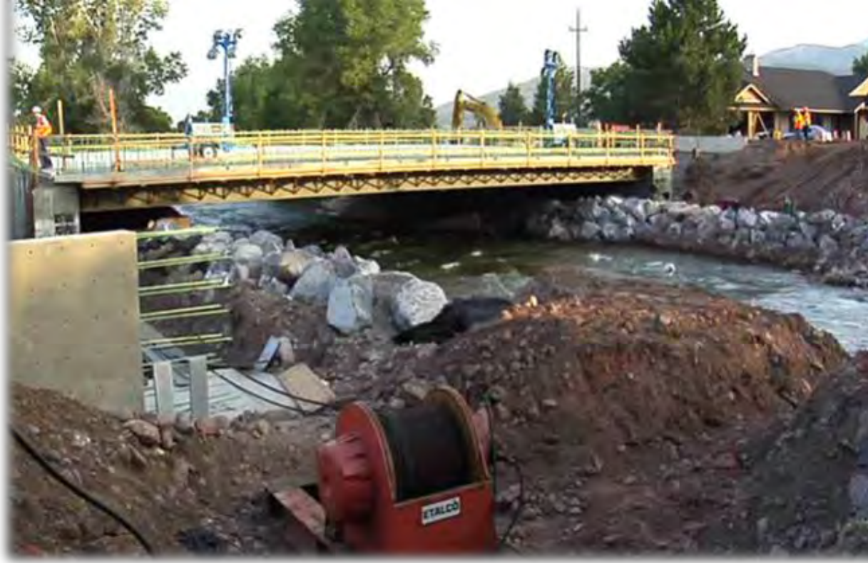
SR-66 over Weber River Bridge Replacement Design-Bid- Build
