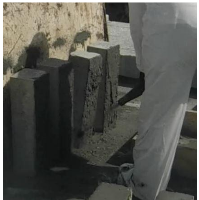
Figure 16. Horizontal Spray note Rebound
