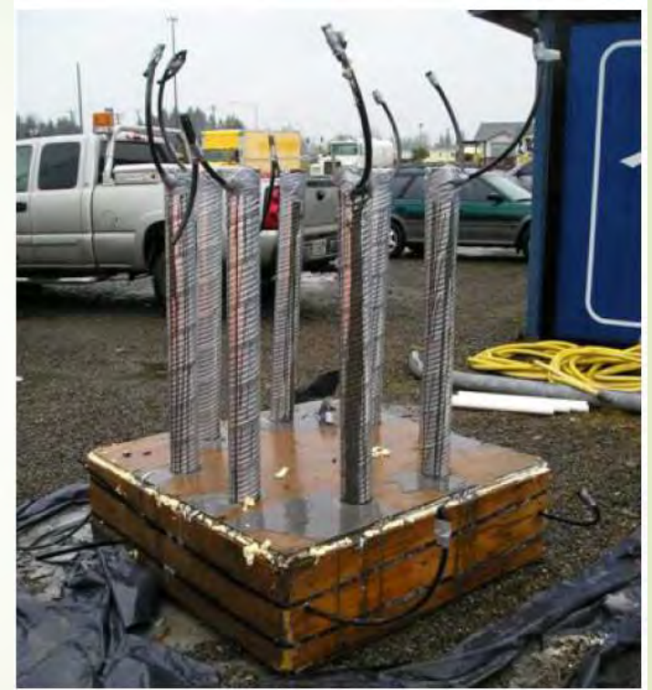
Photo: Mock-up of the grouted joint.
