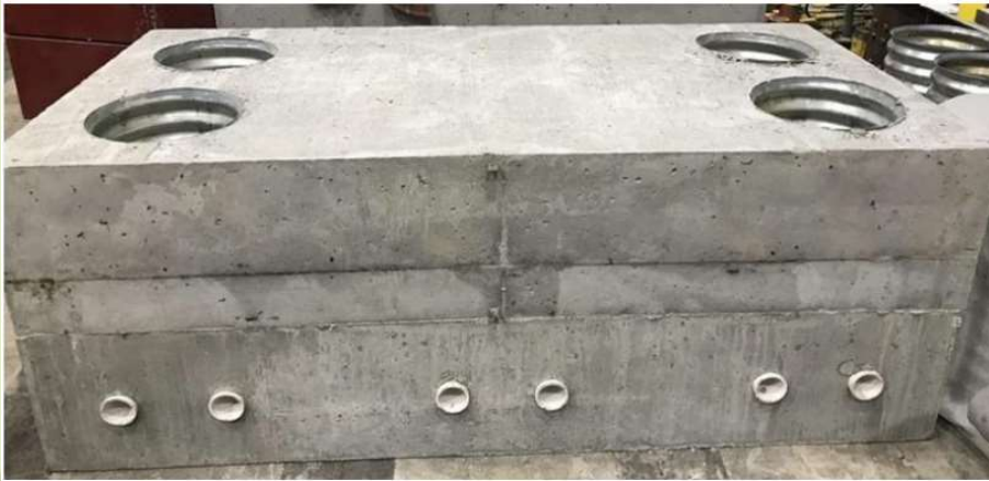
Figure. Bridge cap with pile couplers
