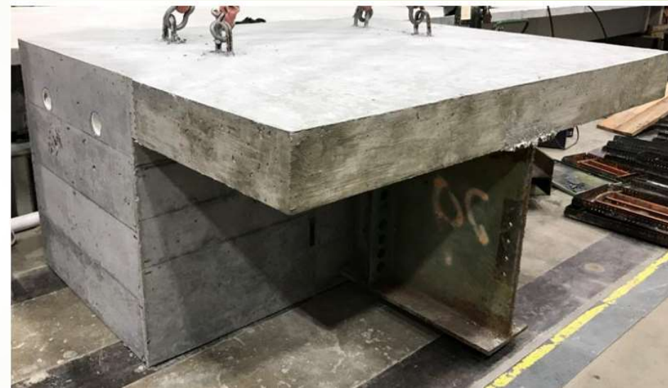
Figure. Pile coupler integral diaphragm completed
