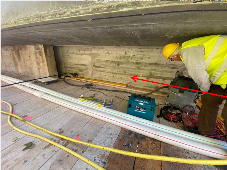
Installation of optical fiber sensor
