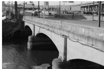
Concrete-encased riveted steel girders
