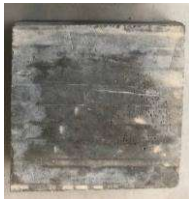
CONCRETE SUBSTRATE BEFORE SURFACE PREPARATION
