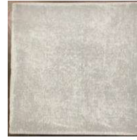
POLYMER CONCRETE OVERLAY AFTER SURFACE PREPARATION
