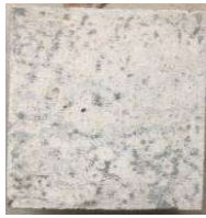
CONCRETE SUBSTRATE AFTER SURFACE PREPARATION
