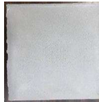
POLYMER CONCRETE OVERLAY BEFORE SURFACE PREPARATION
