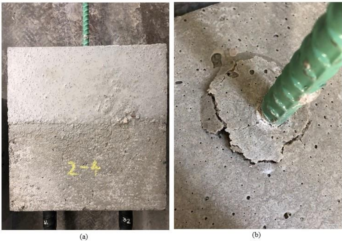
Figure 5-4. (a) Elevation view of pullout failure, 2-04, (b) Pullout at top of HCSC, 2-04
