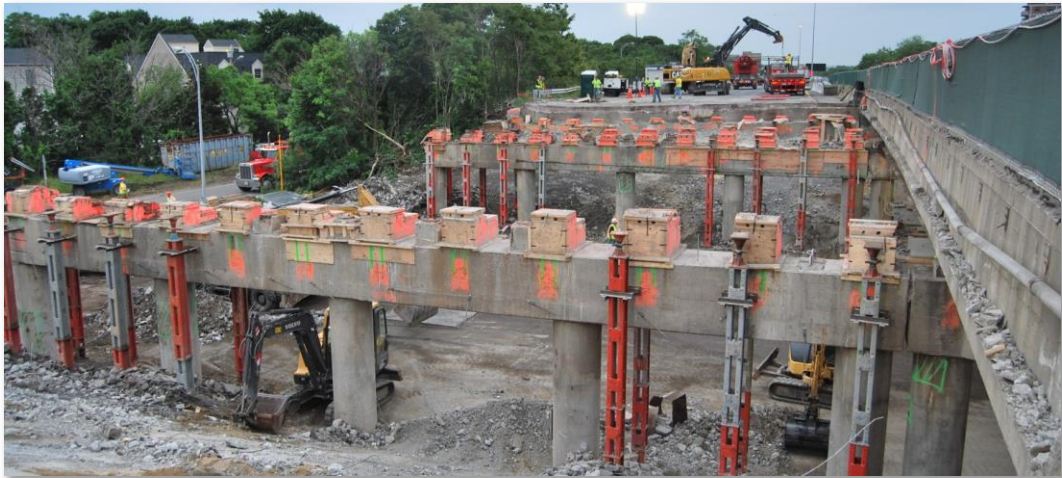
Saturday Morning, 7:00 am – Demolition Complete
