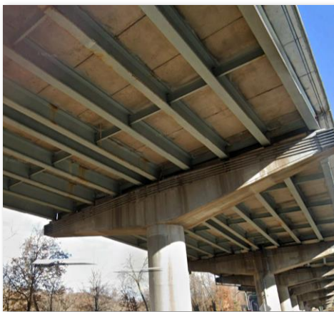
Bridge 00588 deck condition 30 years in service
