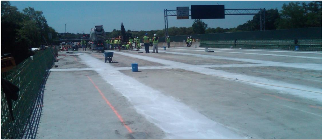
Sunday Morning – Curing of Closure Pours
