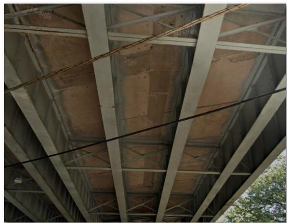
Bridge 00587 deck condition 30 years in service
