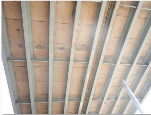
Precast panels 30 years in service
