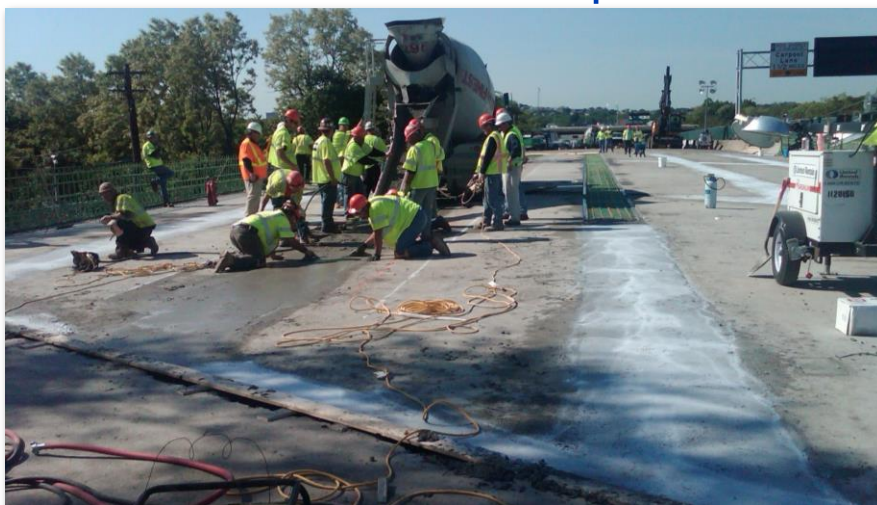
Sunday Morning – Placement of High Early Concrete
