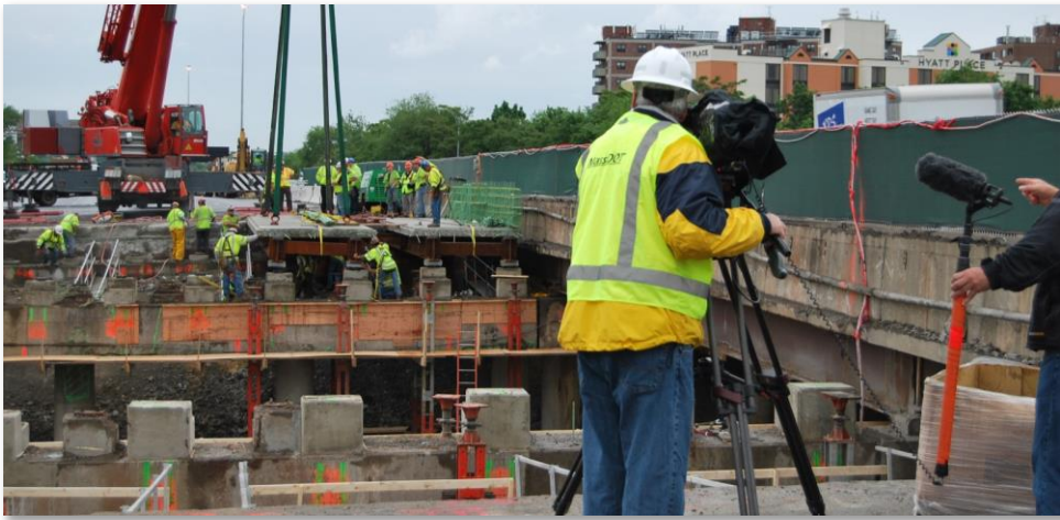
Saturday Morning, 11:30 am – Erection Begins
