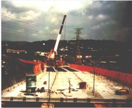
Deck panel erection
