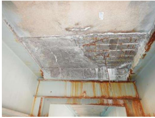
CIP closure pour at leaking deck joint 30 years in service
