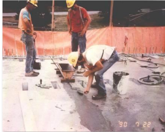
Grouting shear keys
