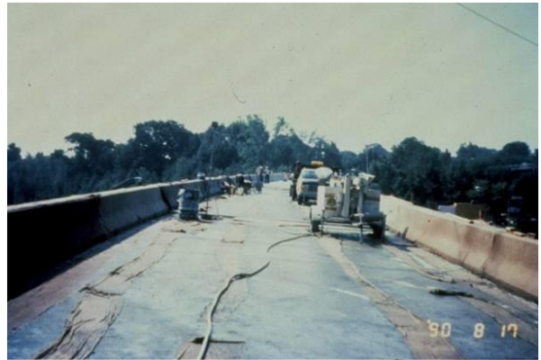
Grouted shear connector pockets CIP parapets
