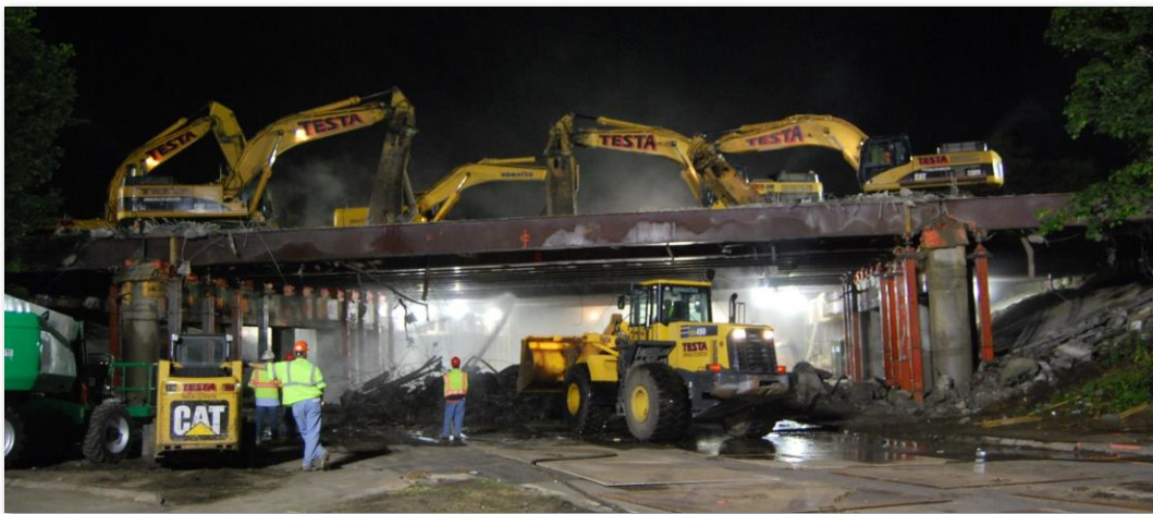
Friday Night, 10:00 pm – Demolition Begins
