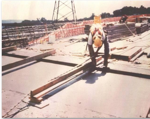
CIP closures at joints
