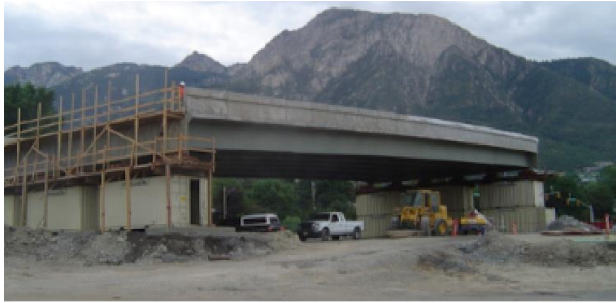
(a) Construction of a bridge using SPMT installation
