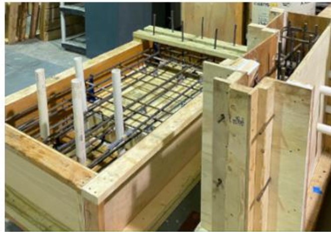
(a) Barrier and deck reinforcement
