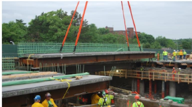
(b) Modular construction of bridges with and without integral barrier
