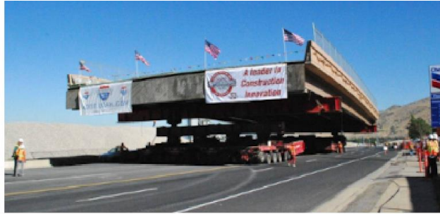
(a) Construction of a bridge using SPMT installation
