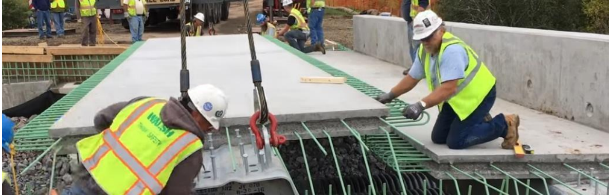
Figure 2 Modular construction with barrier system incorporated into the exterior module.
