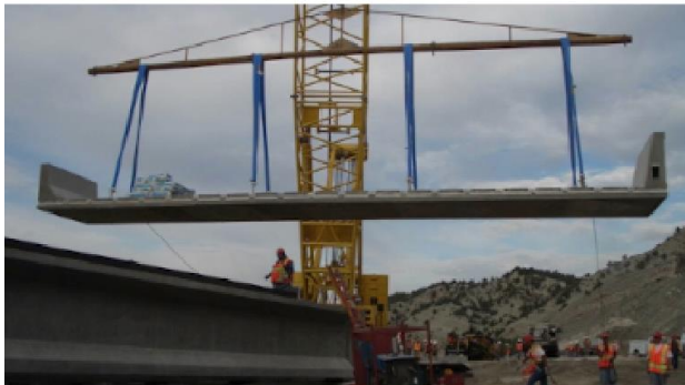
(b) Modular construction of bridges with and without integral barrier
