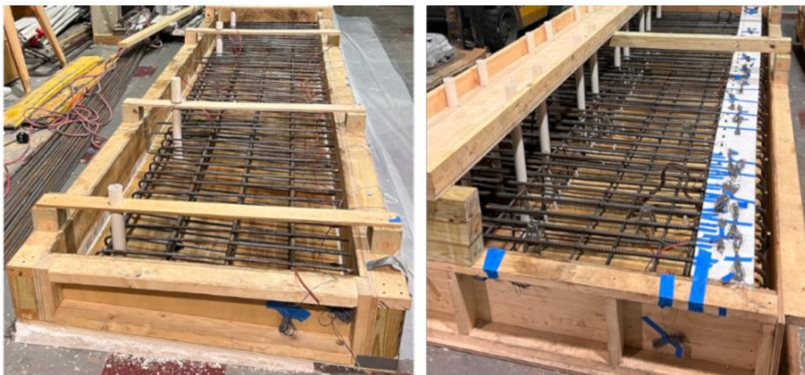
(a) Barrier and deck reinforcement
