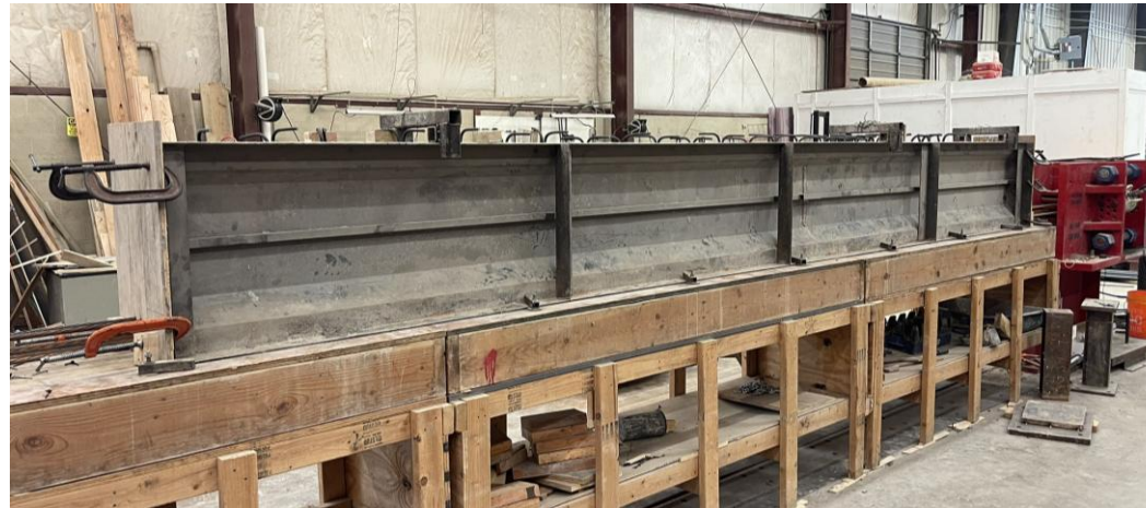
Completed Girder Specimen Formwork
