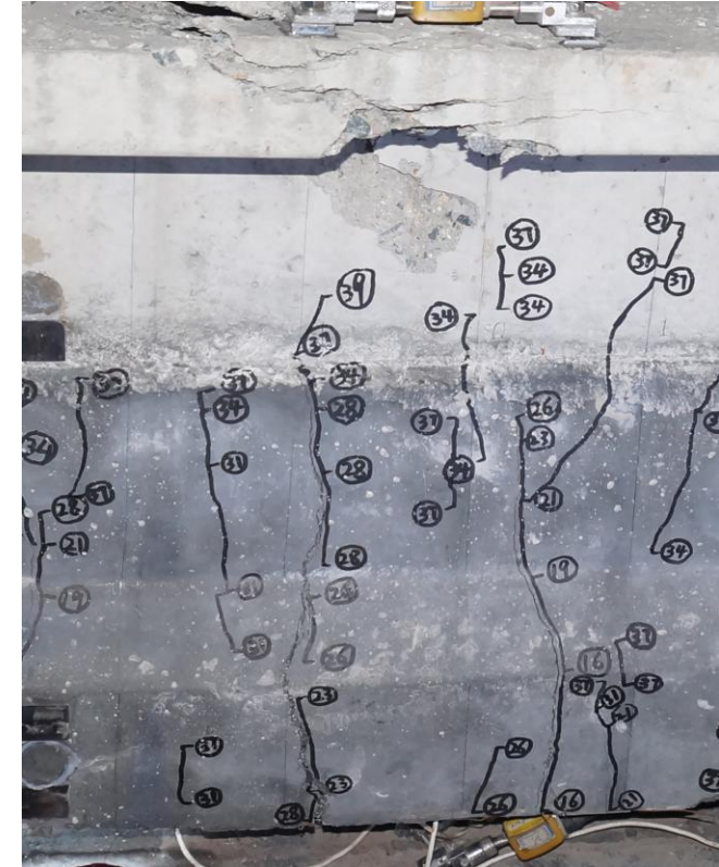
UHPC to Conventional Concrete Interface after Testing (Li et al. 2020)
