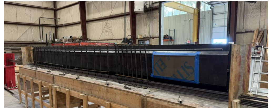
Formwork Side with 3 ft Web Insert and Reinforcement in Place
