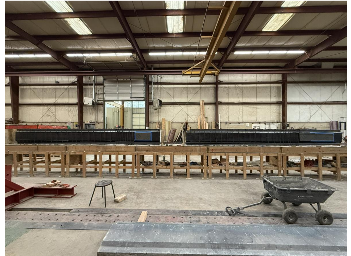
Hybrid Girder Specimen Layout on Prestressing Bed
