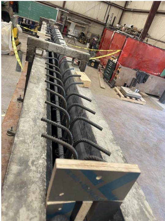
SCC-UHPC Divider in Formwork
