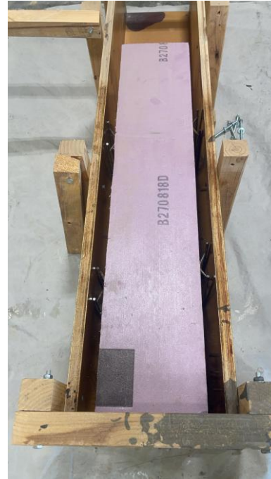
Formwork for Smooth Interface Shell
