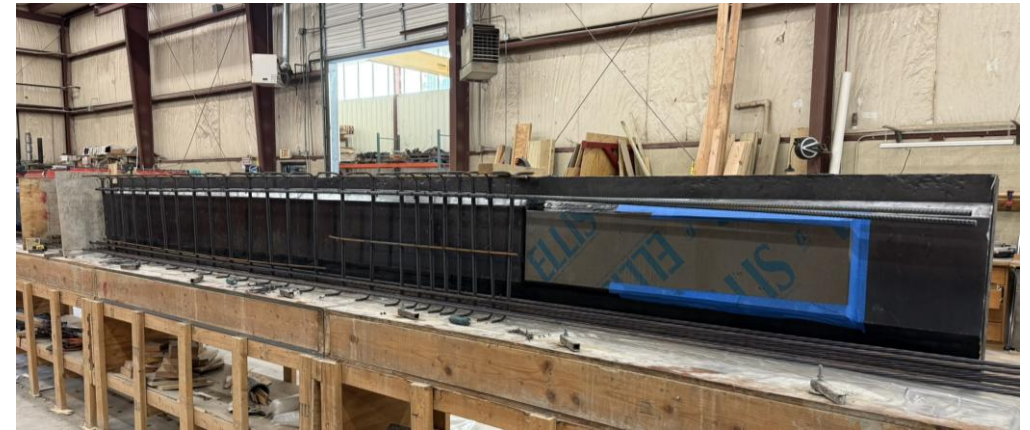
Formwork Side with 5 ft Web Insert and Reinforcement in Place
