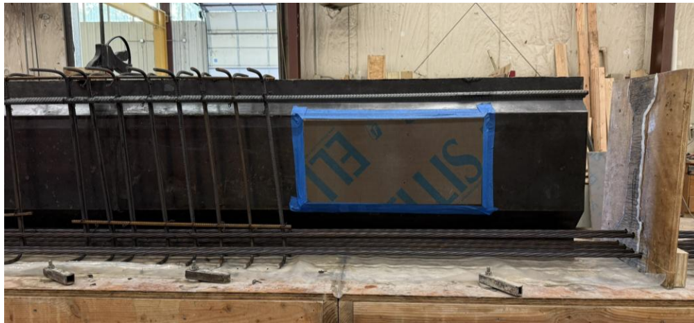
Close-up of 3 ft Web Insert with Reinforcement in Place
