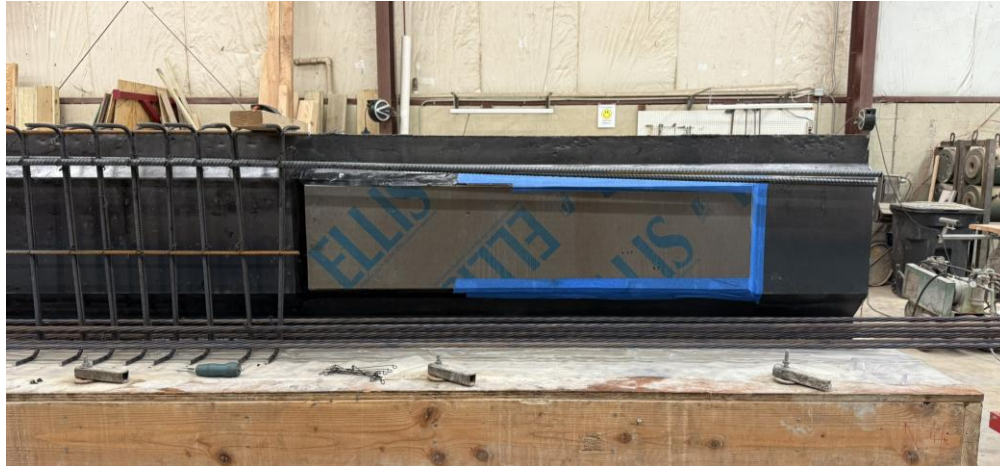
Close-up of 5 ft Web Insert with Reinforcement in Place
