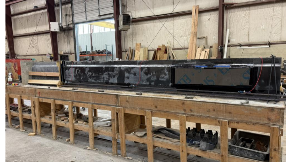
Formwork Side with UHPC Girder Reinforcement in Place
