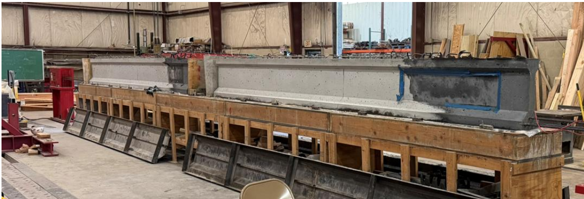
Figure 6. Completed hybrid girder specimens
