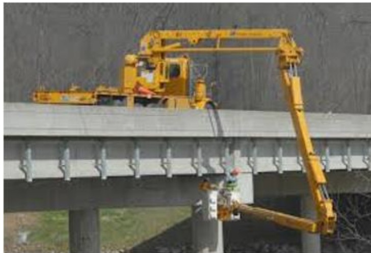
Figure 1: Example of technique currently used to inspect bridges
