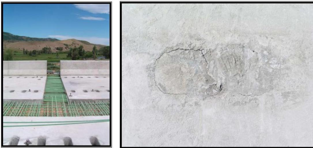
Figure 9: Shrinkage crack in the blockout type of ABC closure joint [13]
