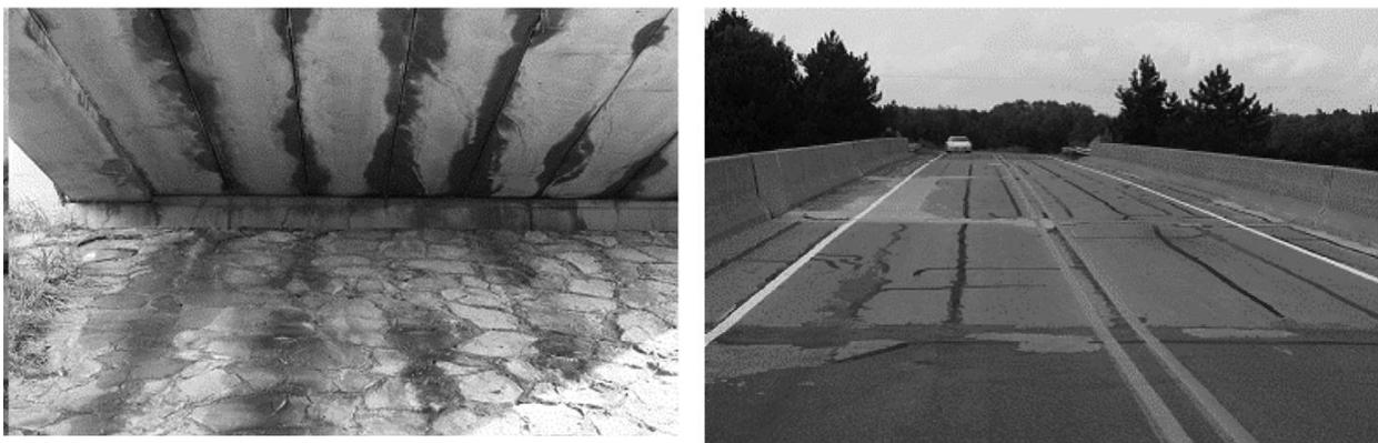
Figure 10: Longitude deck cracking of ABC closure joint [14]
