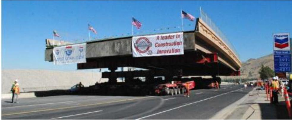
Figure 1: ABC superstructure positioning [5]
