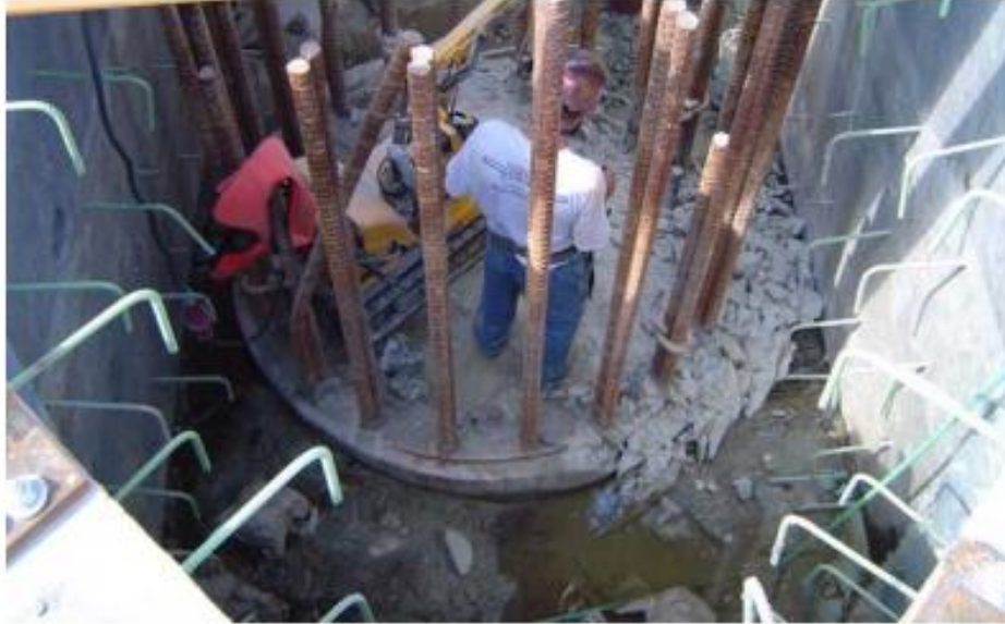
Figure 7 Footing Reinforcing Placement in Providence River Bridge Pier Box
