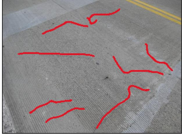
Fig. 18: Multiple Random Cracking in Precast Panel
