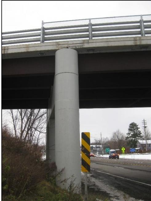
Fig. 9: Precast Pier Cap/Column Connection
