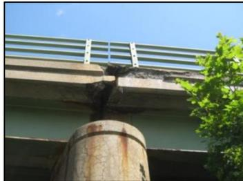
Fig.2: Leaky Joints (7)
