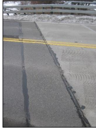
Fig. 23: North Abutment Expansion Joint
