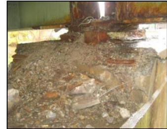
Fig.3: Deteriorated Pedestal (7)
