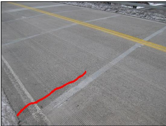
Fig. 19: Parallel Cracks to UHPC Connection
