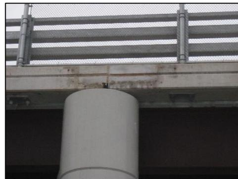
Fig.12: Installed UHPC Link Slab
