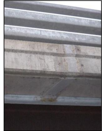
Fig 21: Transverse Joint
