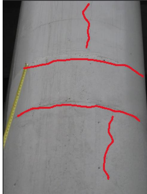
Fig. 10: Vertical Cracks in Column & Pier Cap
