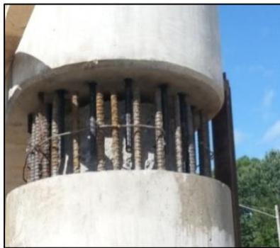
Fig. 6: Rebar Connection
