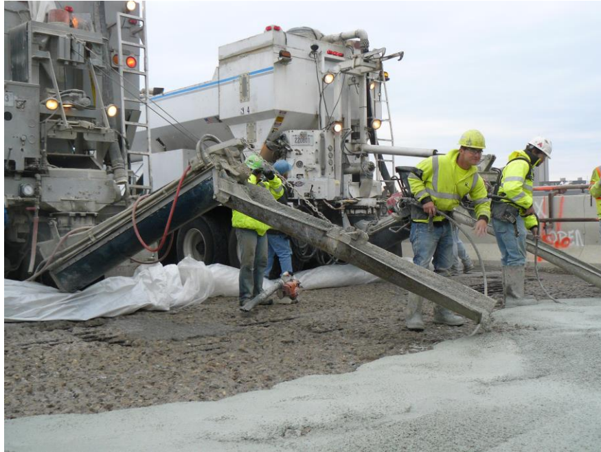
VESLMC being placed on a Fast Track Hydrodemolition Prepared Surface
