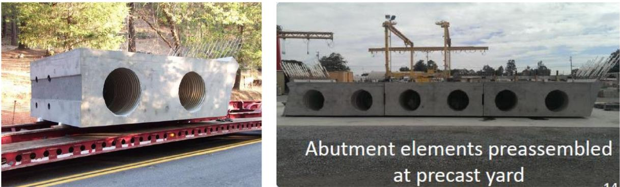
**Fig. 2** – Precast abutment segments for Fort Goff Creek bridge in California (photos are courtesy of Dorie Mellon as adopted from Caltrans ABC-UTC seminar)
