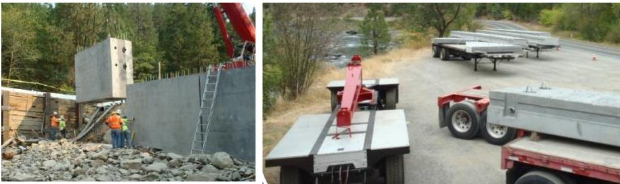
**Fig. 3** – Wingwalls and abutment assembly (left) and deck precast segments (right) for Fort Goff Creek bridge in California (photos are courtesy of Dorie Mellon as adopted from Caltrans ABC-UTC seminar)
