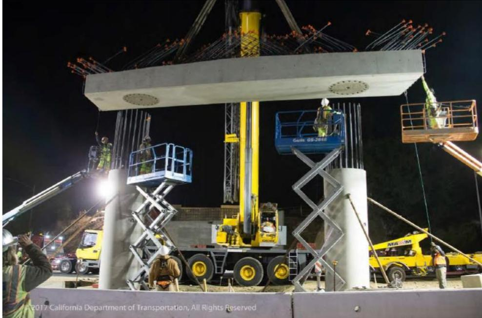
**Fig. 4** – Precast columns and drop bent cap for Laurel Street Overcrossing project in California (photos are courtesy of Dorie Mellon as adopted from Caltrans ABC-UTC seminar)
