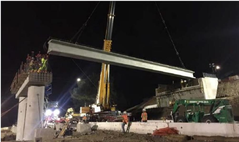
**Fig. 5** – Installing a precast girder for Laurel Street Overcrossing project in California (photos are courtesy of Dorie Mellon as adopted from Caltrans ABC-UTC seminar)
