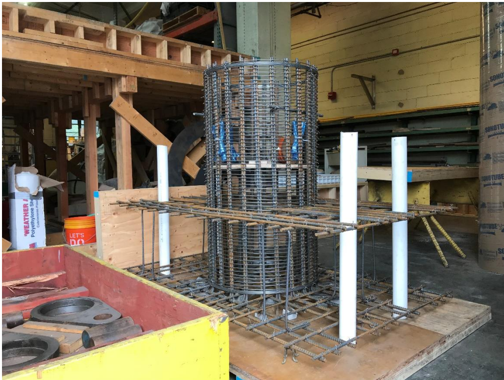
Figure 2. Photo of Specimen Under Construction
