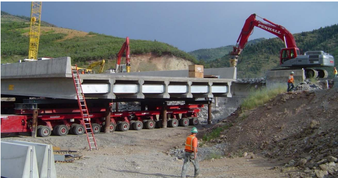
SPMT Bridge System Utah DOT
