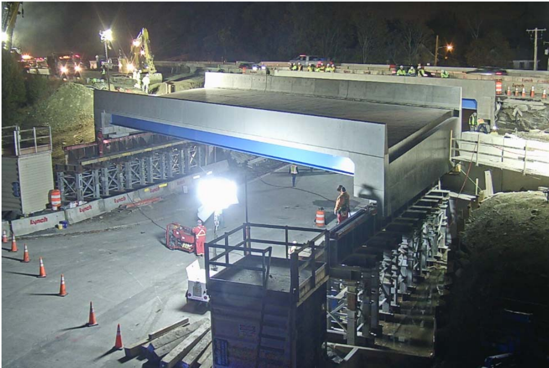
Lateral Slide System Rhode Island DOT
