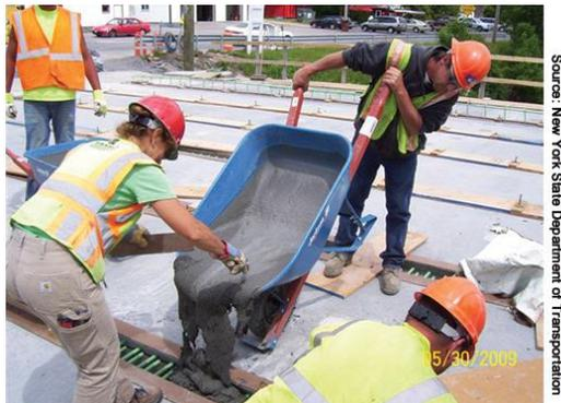
**Figure 4. UHPC being placed into an expansion joint (NYSDOT)**
